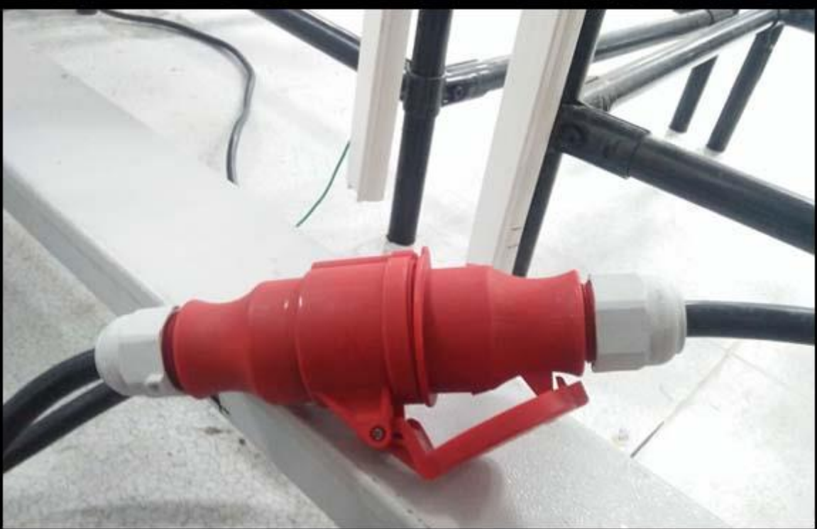
Industrial Plug & Socket Connection - Three Phase
