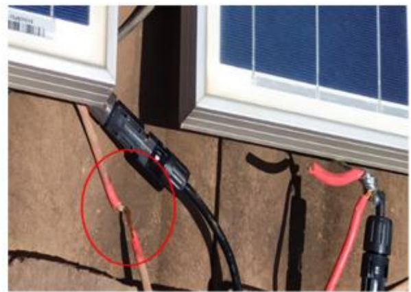
b. Animal bites on a wire of 5-year old solar PV system in Dry Equatorial Climatic Zone
